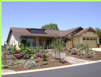
Danielsen Construction & Energy Mgmt. 807 Smith Flat Rd Angels Camp, CA 95222 (209) 728-4921
